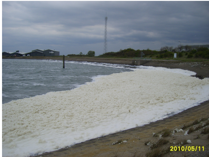
Figure 8.3. Open intake of the Jacobahaven plant, showing the foam caused by algae.
